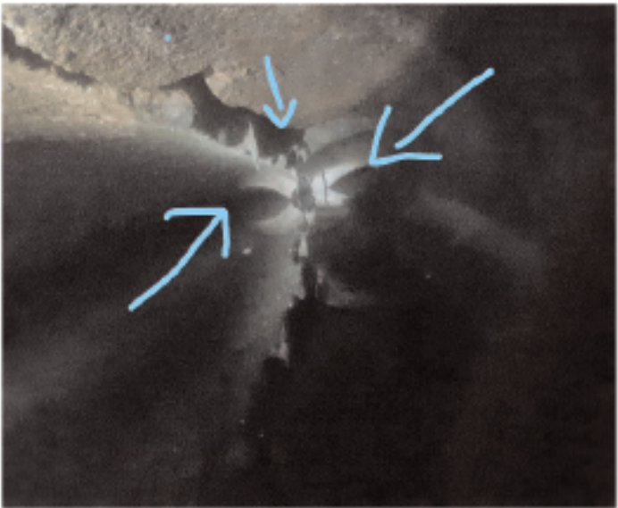
Area within the sewer that is collapsing.
