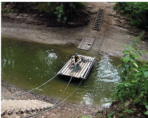
Rope Pull Channel Crossing
